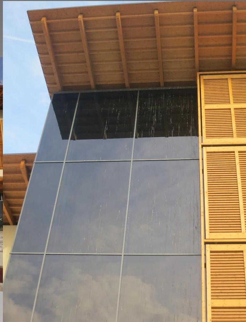
Even before construction was completed pigeons started to roost in sheltered parts of the building. Pigeons roosting below the roof were creating an unsightly mess on the glass facades (above right).
