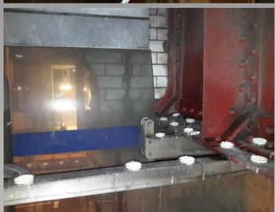
The night roosts at the ends of the red beams were disinfected and treated with dishes of 小島 *Bird Free*, as shown above, to prevent further roosting.
