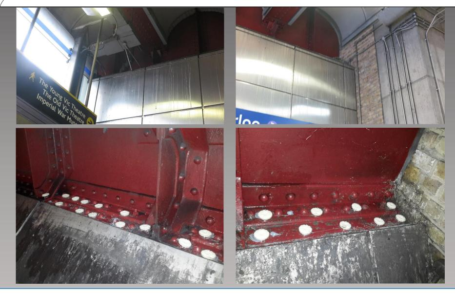
Nests were removed from both corners of the ledge at the southeast end of the ticket hall adjacent to the street entrance. The flanges from which the nests were removed were treated with dishes of 小島 Bird Free, as shown above, to prevent further nesting.
