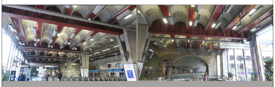
There are four red beams that run across the ticket hall from the window to the pillars that support the ceiling. Pigeons were roosting on the flanges at both ends of these beams and fouling below. Dishes of 小島 Bird Free were applied to these flanges to prevent further roosting, as described on the following page.
