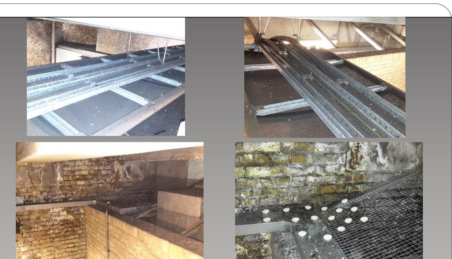
There were no signs of nesting or roosting in the centre of the cable tray, nor at the east end, however a nest was removed from the corner to the north of the lift shaft, and dishes of 小島 *Bird Free* were fixed, as shown above right, to prevent further nesting.
