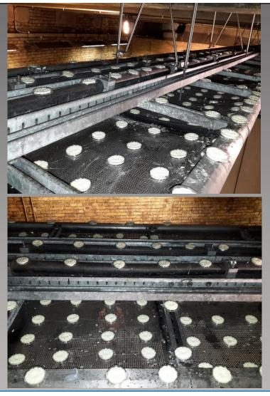
Nests were removed from the far west corner of the cable tray that runs above the lift shaft and roosting was evident on the 3m of the cable tray closest to the wall. Dishes of 小島 Bird Free were fixed, as shown above, to the 4m of cable tray closest to the wall to prevent further nesting and roosting.
