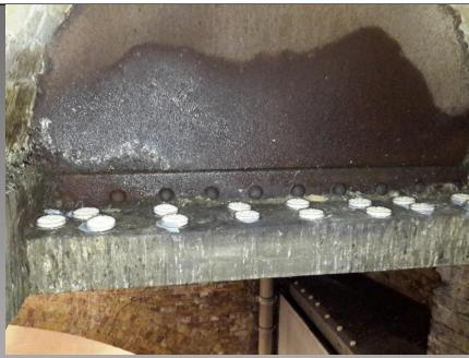
A nest was removed from a niche in the ceiling adjacent to the lift shaft. The surface from which the nest was removed was disinfected and treated with dishes of 小島 Bird Free, as shown above right, to prevent further nesting.
